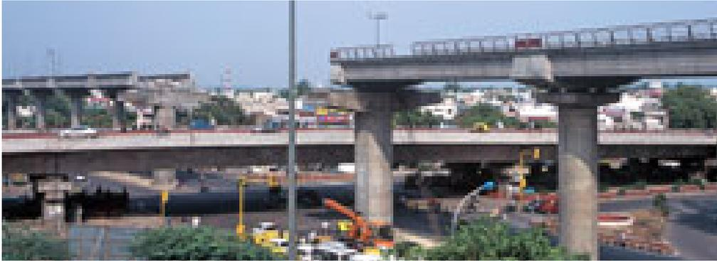
drains. Due to the highly acidic underground water of Delhi, slag cement was used for pile concrete.
